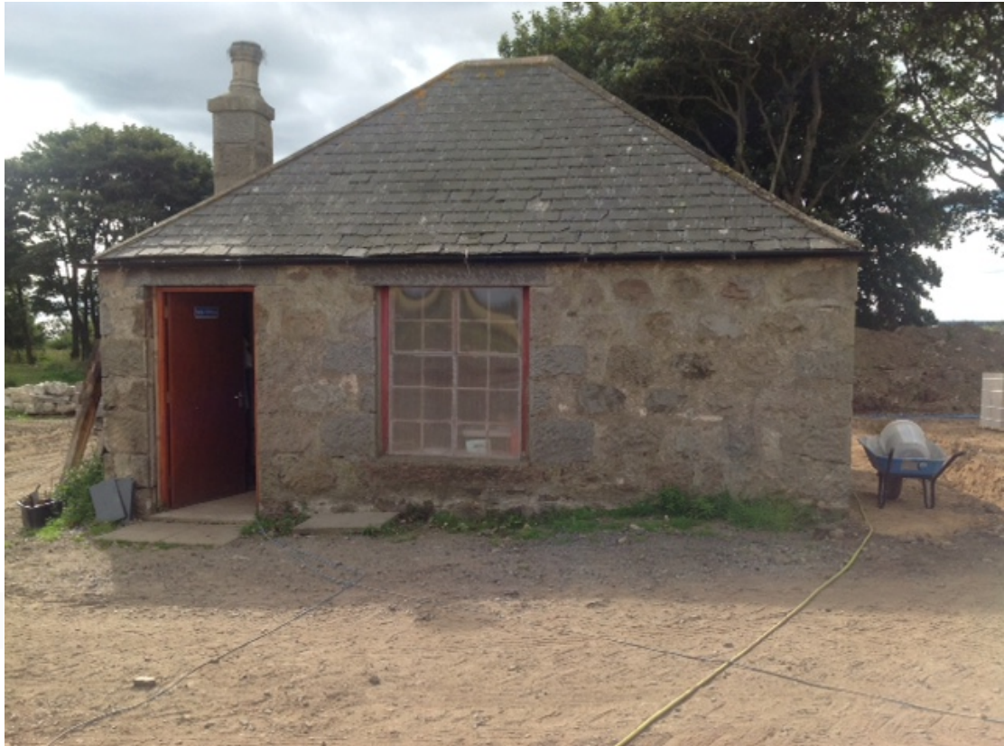
Fig.1 Existing Bothy, Sleeping Accommodation
