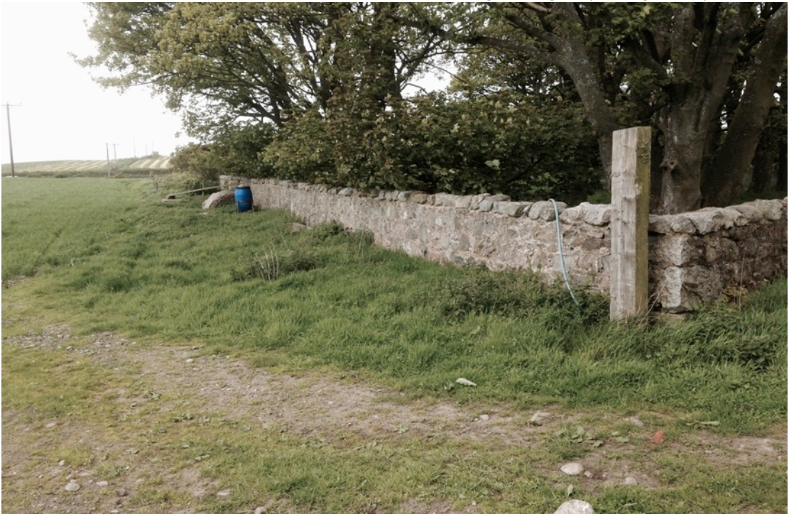
Fig.7 Existing South Boundary, Existing Stone Dyke to remain Boundary Trees to remain to maintain border to Green Space Network
