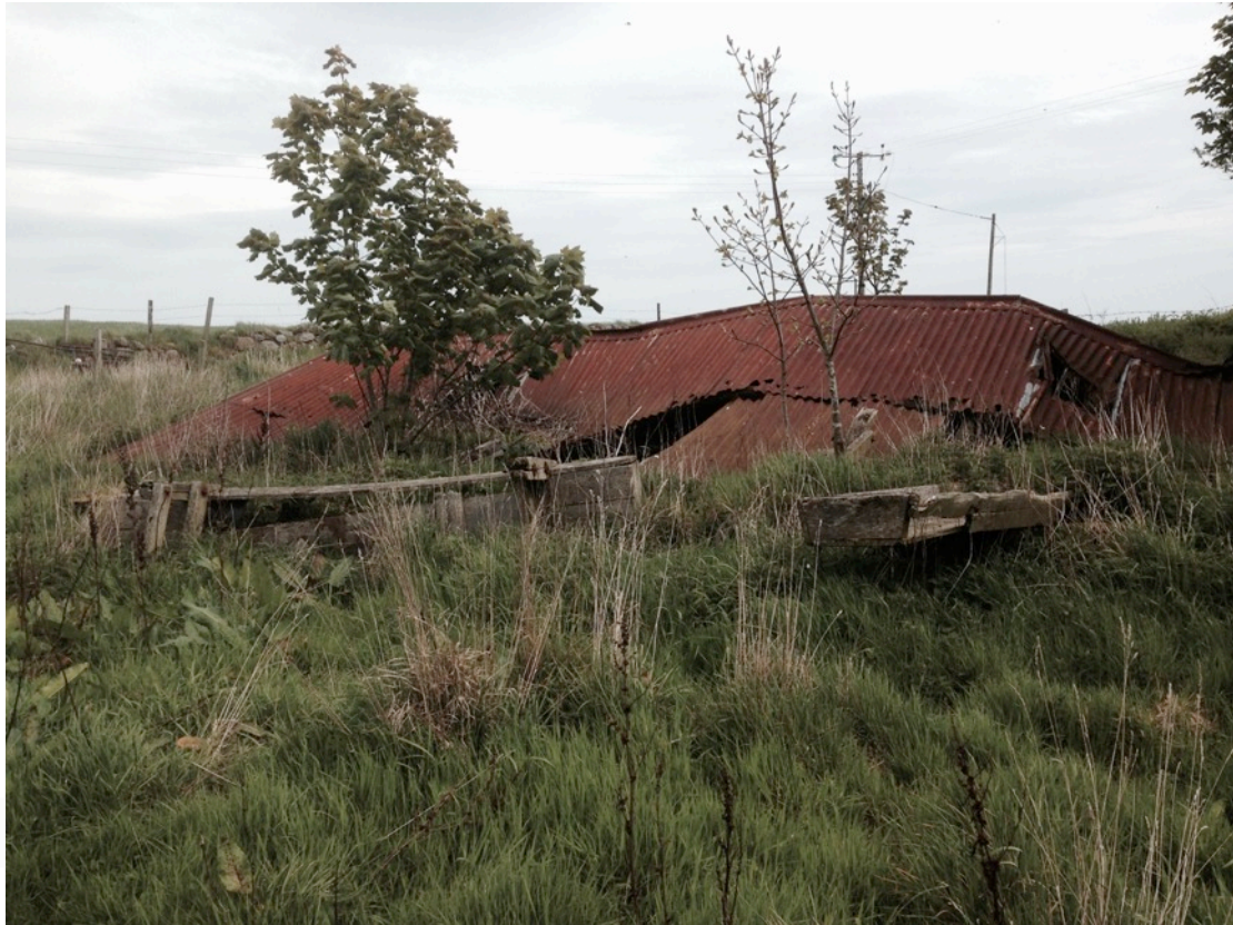
Fig.4 Dismantled shed to East of site.
